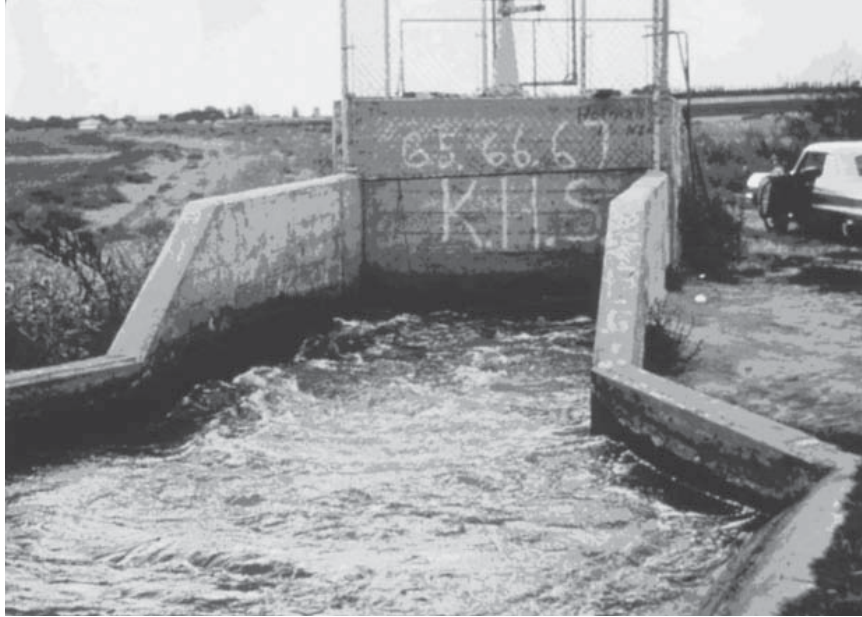
FIGURE 2-1 “The bubbles.” The depth of the water at this point was 2.1 meters, the walls rose 1.1 meter above the water and were 3 meters apart. The churning of the water was caused by subsurface feeding.
